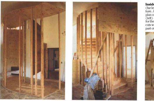
**Inside the staircase.** Assembly of the stair (far left) starts with a plywood and stud armature. A pair of plywood patterns defines the plan of the stair (drawing below). Pairs of studs (left) carry 2x12 cross ties that serve as risers for the stair. Blue tape (below) shows where the cuts were made to remove everything that's not part of the finished stair.
